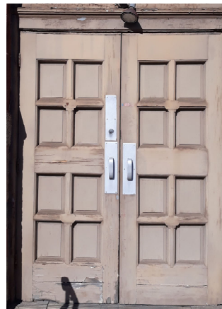
Current Frontage Rd. door.
